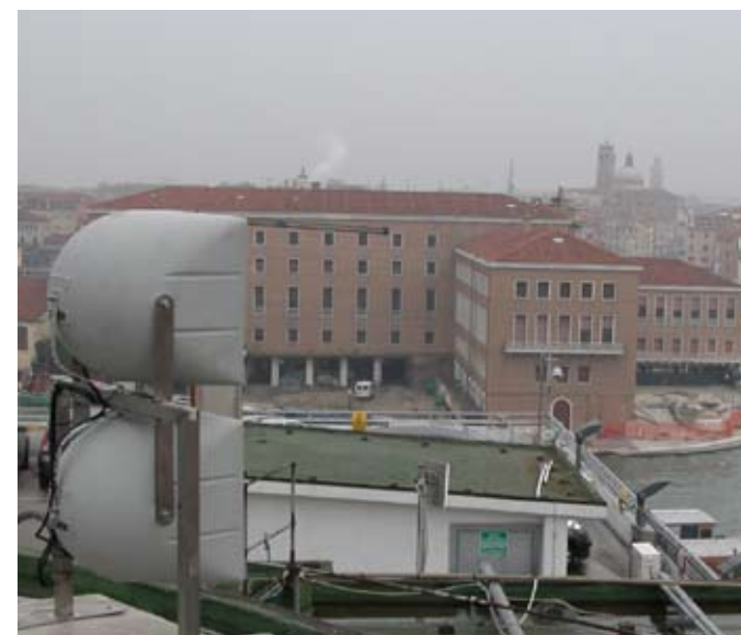
R.5 loudspeakers are strategically placed around the city of Venice as part of its flood warning and evacuation system.
